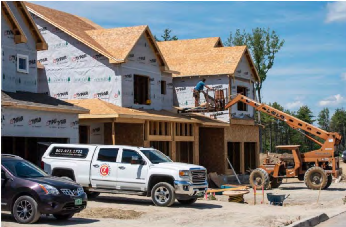
Construction underway on new homes at the Hillside at O'Brien Farm development in South Burlington on Monday, June 22, 2020. Costs of lumber and building supplies have shot up during the pandemic. Glenn Russell/VTDigger
